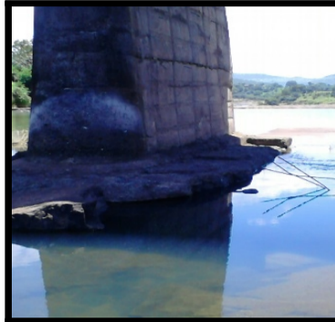
Plate 10: Present scene of Bridge Pier foundation exposed due to scouring of rocks at Chaskaman Dam side spillway (Nov.2013)
