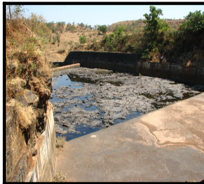
t █ ۞ ۞ The bed concrete apron protection wall adopted just near the Spillway location
