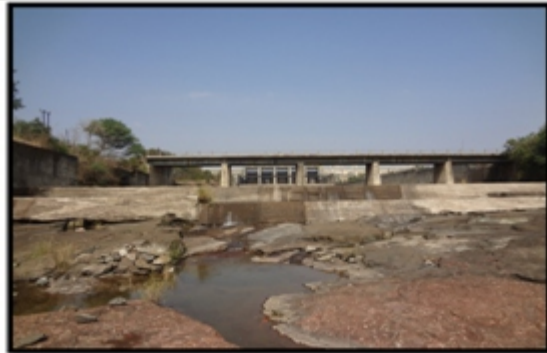
Plate 12. Guide bund provided at the downstream of bridge to control velocity of flow as well as future rock scouring in river portion (2009)
