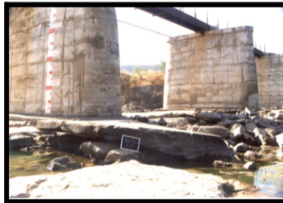
Bridge Pier foundation exposed due to scouring of rocks at Chaskaman Dam side spillway (2001)
