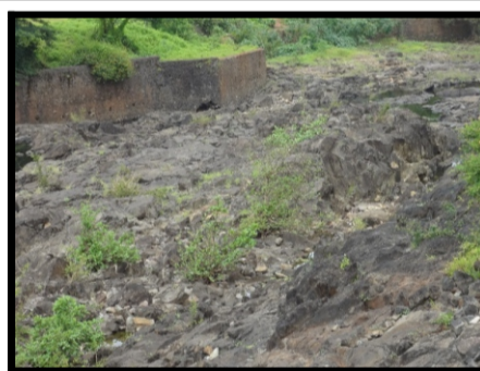
t █ ۞ ۞ Deep Gullies formation process occurring in the spillway channel.
